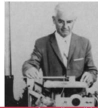
The rectilinear scanner for radionuclide diagnostics was created (B. Cassen). For more than two decades the Cassen scanner became the main tool of nuclear medicine
